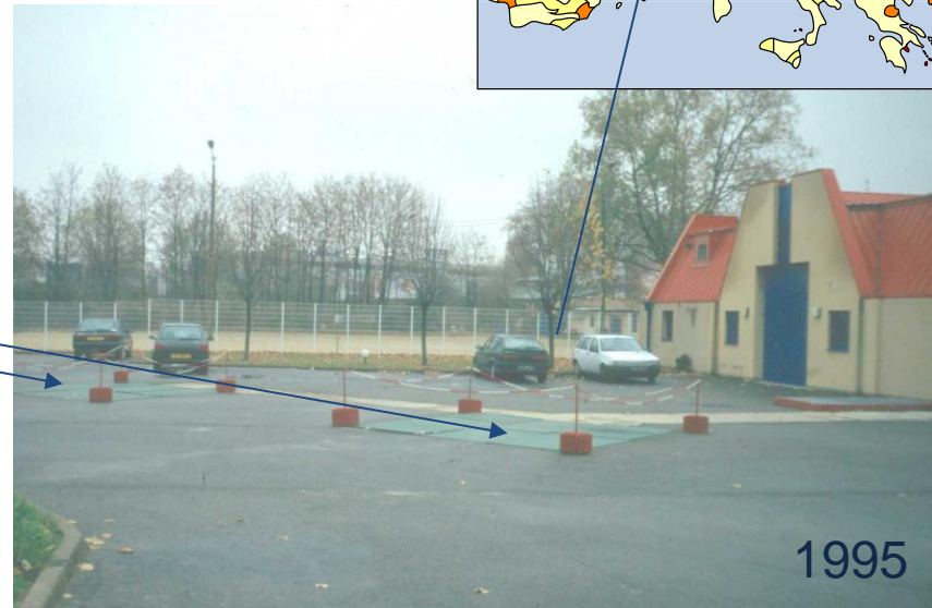
Geothermal central in Chevilly-la-Rue, south of Paris, France
