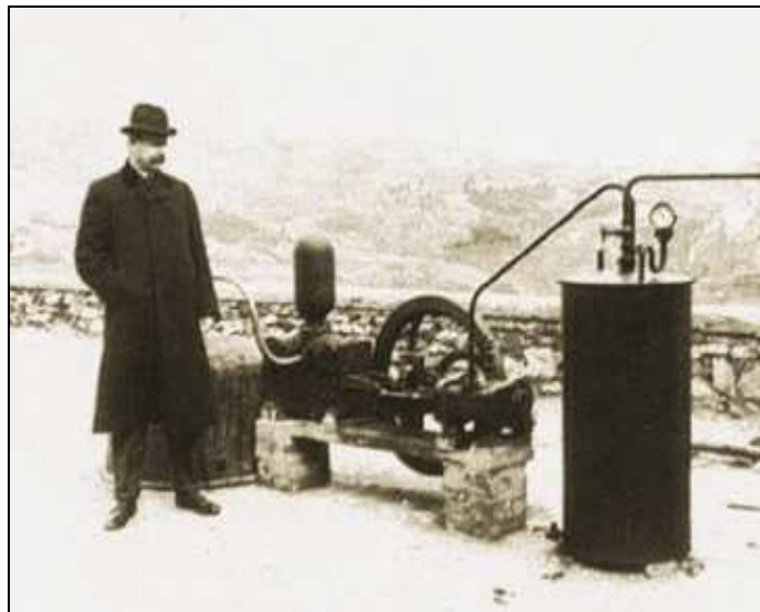
Figure 3. The world's first geothermal power station with a 10kW generator at the Larderello dry steam field, Italy, Tuscany (source: IGA material)
