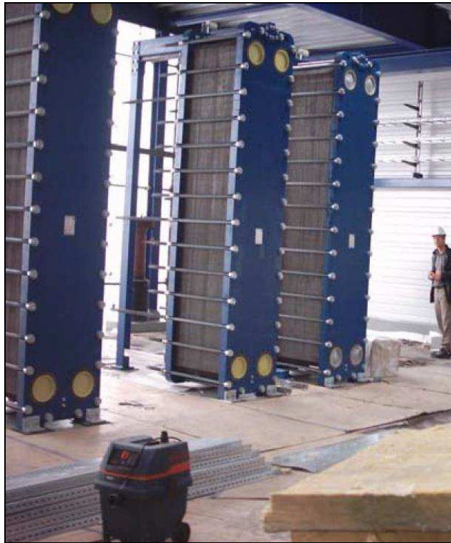
Figure 40. High plate heat exchangers in series ensure an efficient transfer of heat energy from the geothermal water to the district heating water (Lorenzen et al., 2014)
